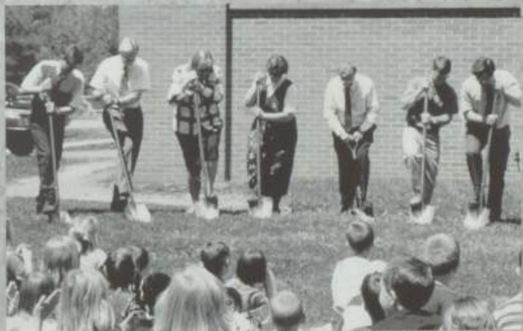
The School Board at Ground-breaking to officially begin renovations of the Elementary School.
